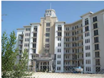
Front of Building
